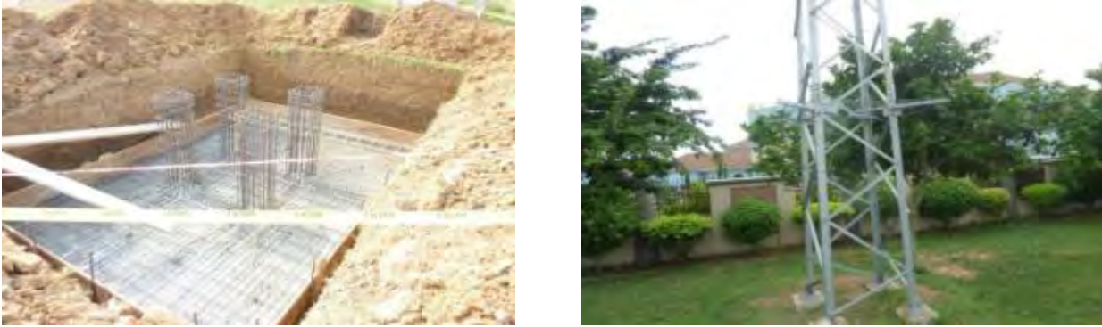
FIGURE 2-4 Foundation Construction and Base of Steel Lattice Tower
