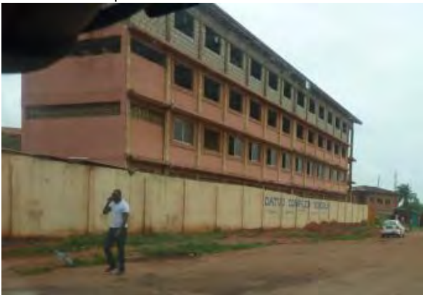
E. Little disturbance as ROW clear (trench on left) but different urban form from photo D
