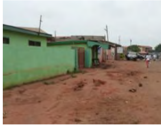
D. Little disturbance as ROW clear (trench on left)
