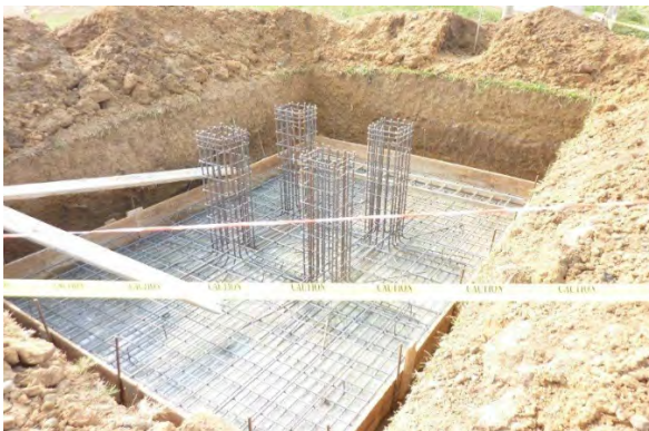
FIGURE 6-3 Foundation Construction and Base of Steel Lattice Tower
