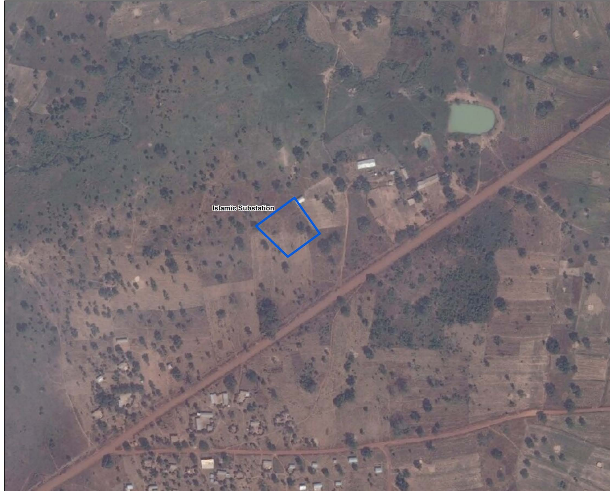
FIGURE 7-7 NEDCo- Engr-09 Islamic Primary Substation Aerial
