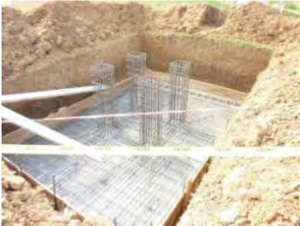
FIGURE 6-3 Foundation Construction and Base of Steel Lattice Tower
