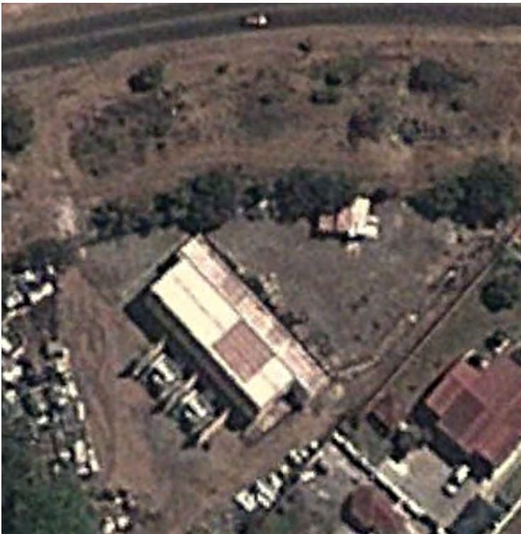
FIGURE 9 Typical indoor primary substation with metal-clad switchgear and underground incoming sub-T
