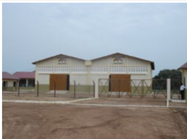
The 1,000 metric tons Warehouse of the Bonyon Agri-Business Centre in the Ejura-Sekyedumase District of the ABZ.
