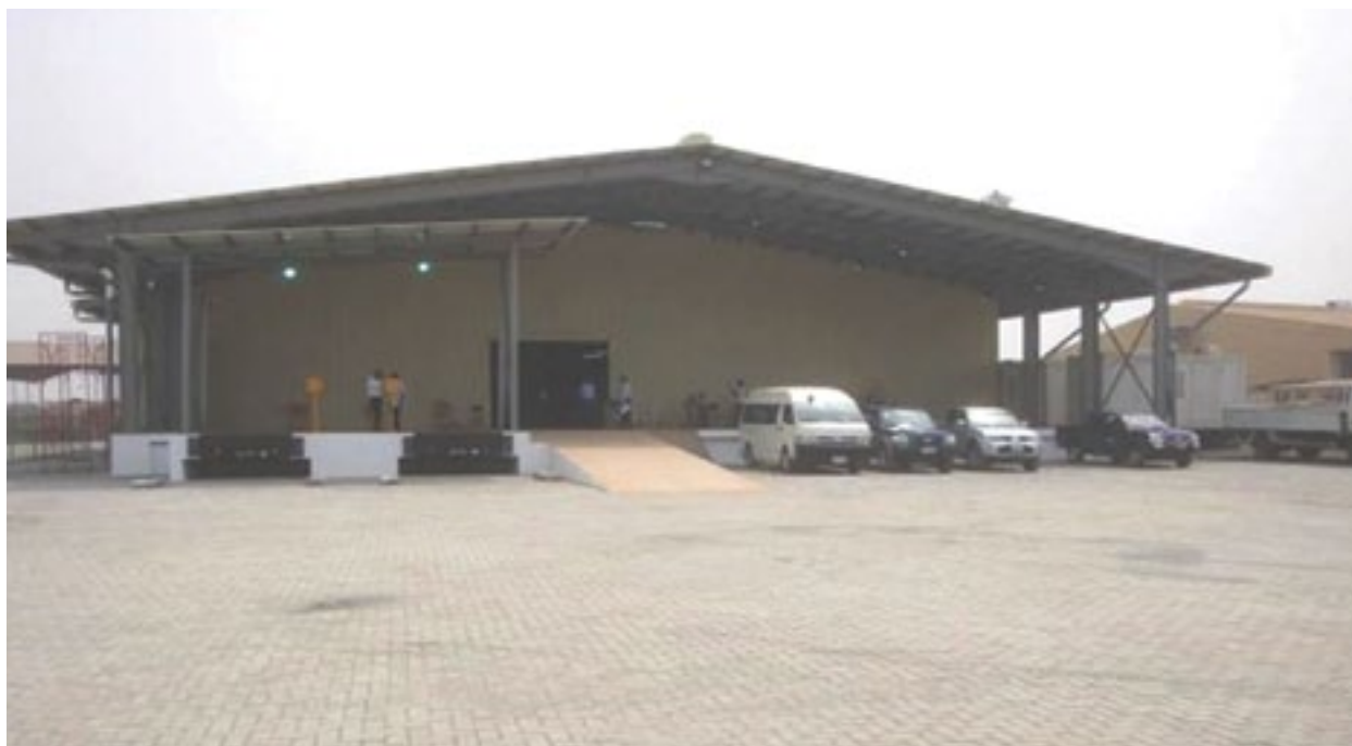
Figure 3.5: PCC at the Kotoka International Airport (KIA)
