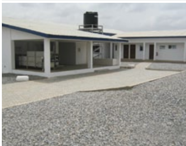
Public Pack-house at Mariakrom in the Akwapim South District of the SHZ West
