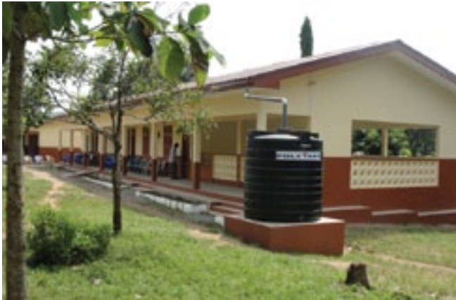
Completed Kindergarten Block, showing Play Area and rain water storage tank at Fotobi in the Akwapim South Municipality
