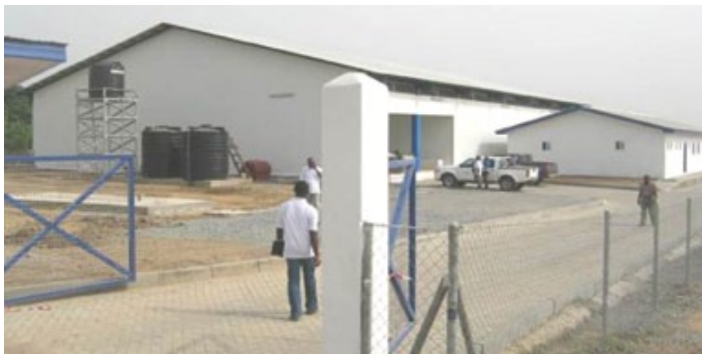
Figure 3.4: The Akorley Pack-house Facility
