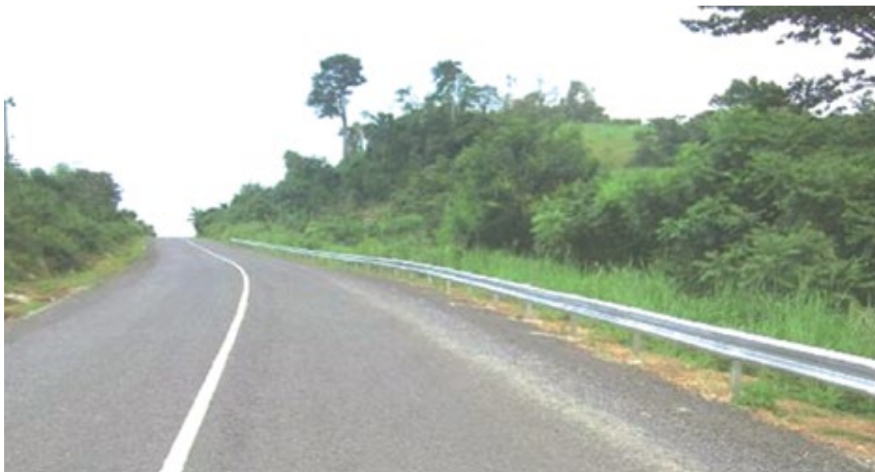
Figure 3.6: Lot 2, EC 1 Contract – Guard Rails on the Odeikrom-Pakro Road - (Ch 4+600)
