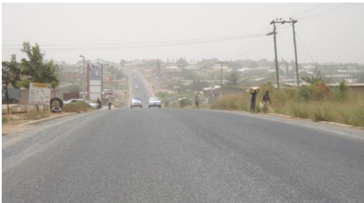
Figure 3.7: A Section of the Upgraded Amanfro–Bawjiase Feeder Road - EC 3
