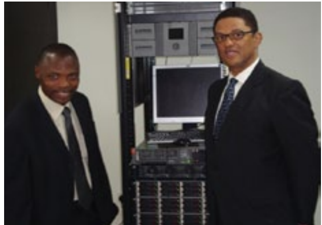
Data Centre equipment being inspected by Apex Bank DMD and an MCC Official.
