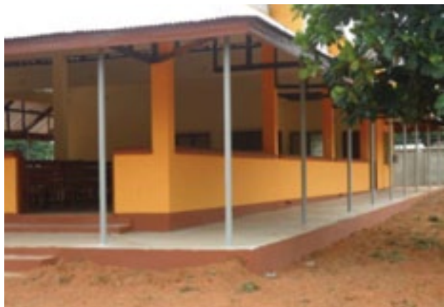
Partial view of the Ferry Terminal at the Adawso end after construction
