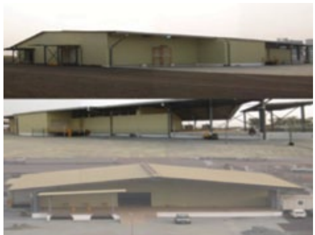
Sides and front views of the Perishable Cargo Center (PCC) at the Kotoka International Airport (KIA).
