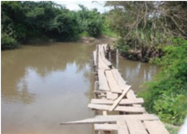
Bridge crossing on the Afrisere-Dome Trunk Road before construction.
