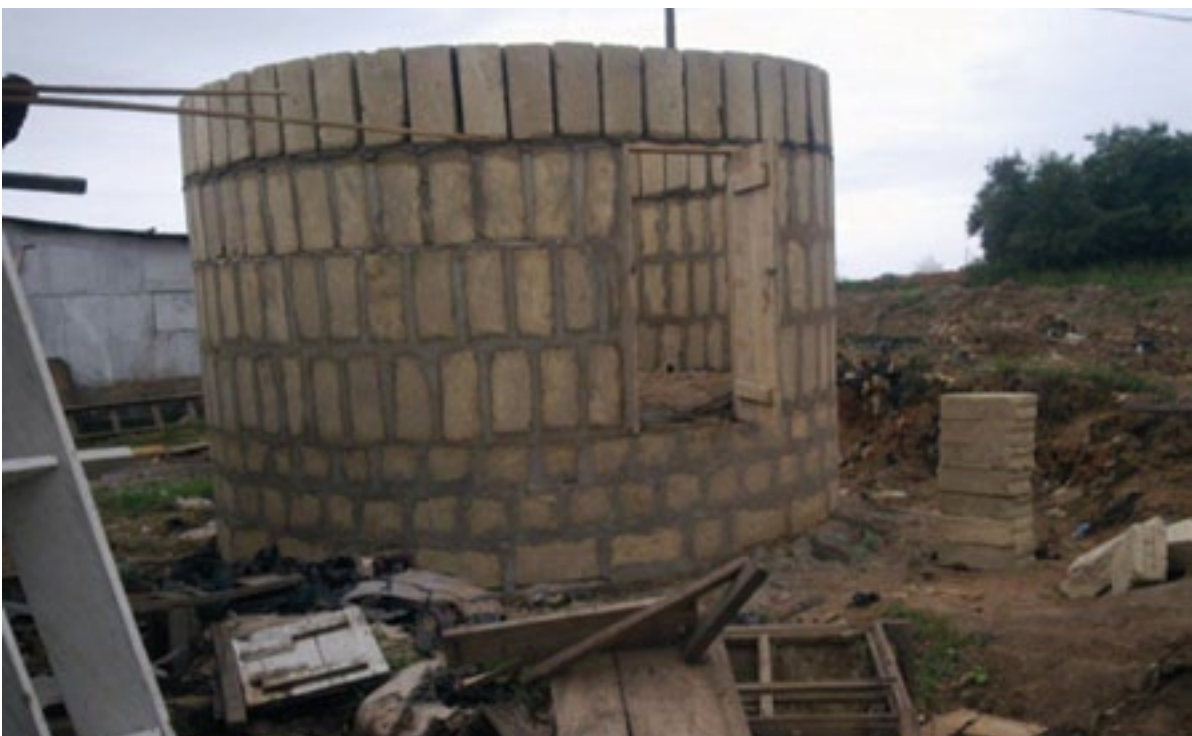
The construction of a relocated Shrine affected by the N.1 Highway.
