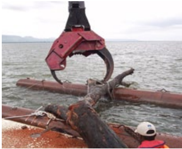
An average tree stump being removed from the navigational path.
