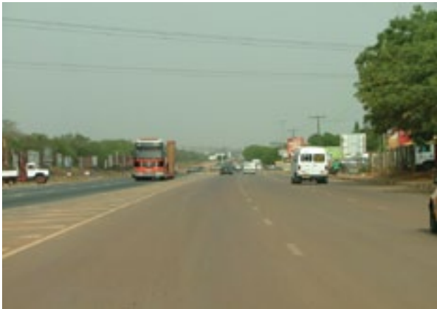
Another section of the N1 Highway Lot 1 – Tetteh Quarshie - Apenkwa at Pre-construction: Before
