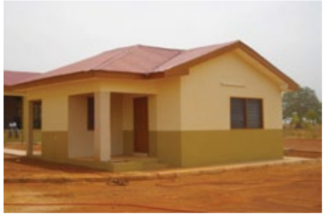
The Administration block of the ABC at Woriboggu-Kukuo in the Tolon Kumbungu District of the Northern Agricultural Zone.
