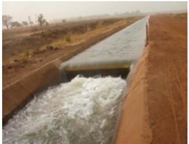
Main Canal Check Structure at Bontanga Scheme: After
