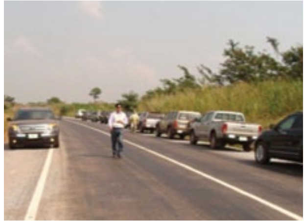
A section of the Agogo-Afrisere Trunk Road after construction
