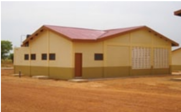
Side view of the Primary Processing Shed of the Woriboggu-Kukuo ABC in the Tolon Kumbungu District of the Northern Agricultural Zone.
