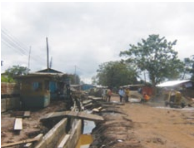
A section of the Kpandu-Kudzra Road in the Volta Region: Pre-construction
