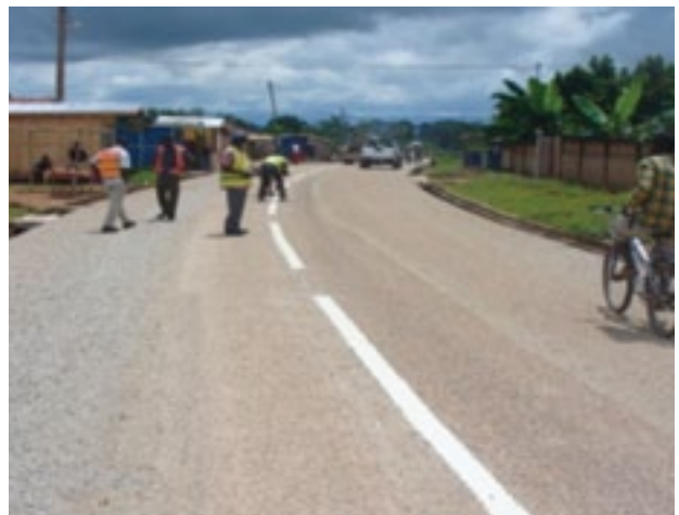
A section of the Kpandu-Kudzra Road in the Volta Region: Post-construction
