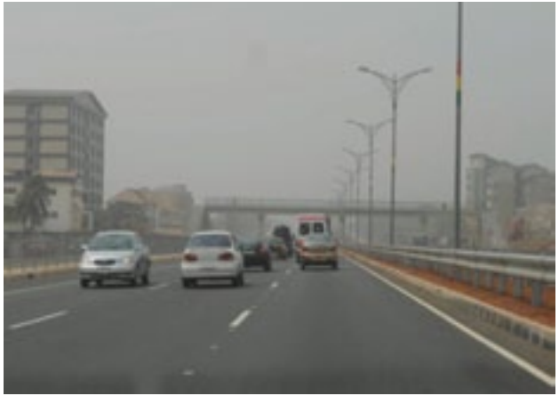
A section of the N1 Highway, Lot 1 – Tetteh Quarshie – at Apenkwa Post-construction: After
