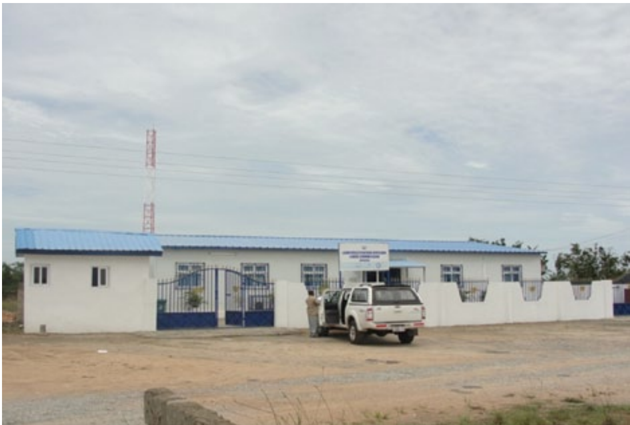
The Winneba Land Title Registration Office. Similar offices were constructed and furnished in Savelugu and Donkorkrom in the Savelugu Nanton and Kwahu North Districts respectively.
