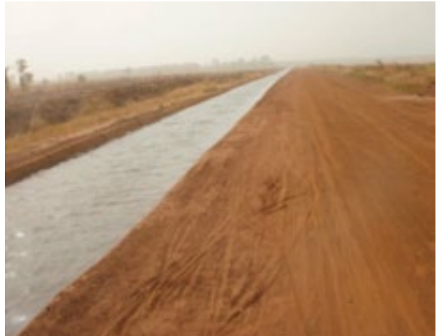
Main Canal Access Roads at Bontanga: After
