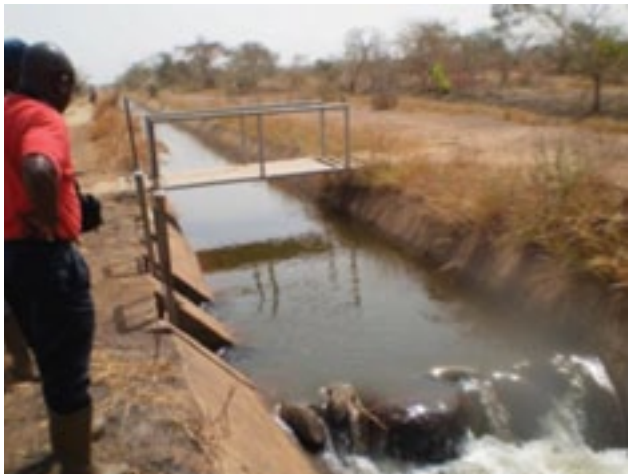
Main Canal Check Structure at Bontanga Scheme: Before
