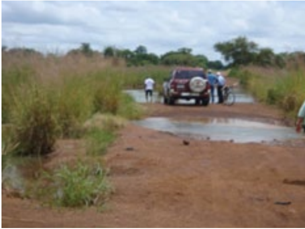
A Pre-construction view of a section of the Savelugu Kpandu Batoyili Feeder Road that suffers perennial flooding in the Northern Region.
