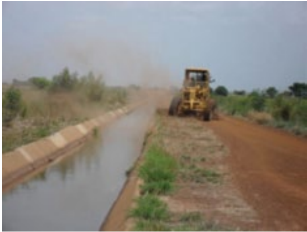
Main Canal Access Roads at the Bontanga: Before
