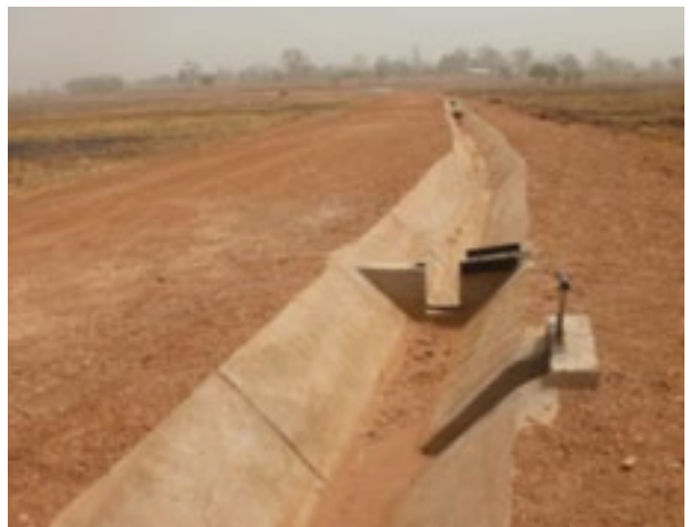
Lateral Canals and Embankments at Golinga Scheme: After
