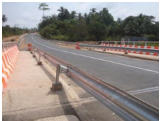
A post-construction view of the Kwanyako Bridge along the Akoti-Desum-Kwanyako Feeder Road in the Central Region.
